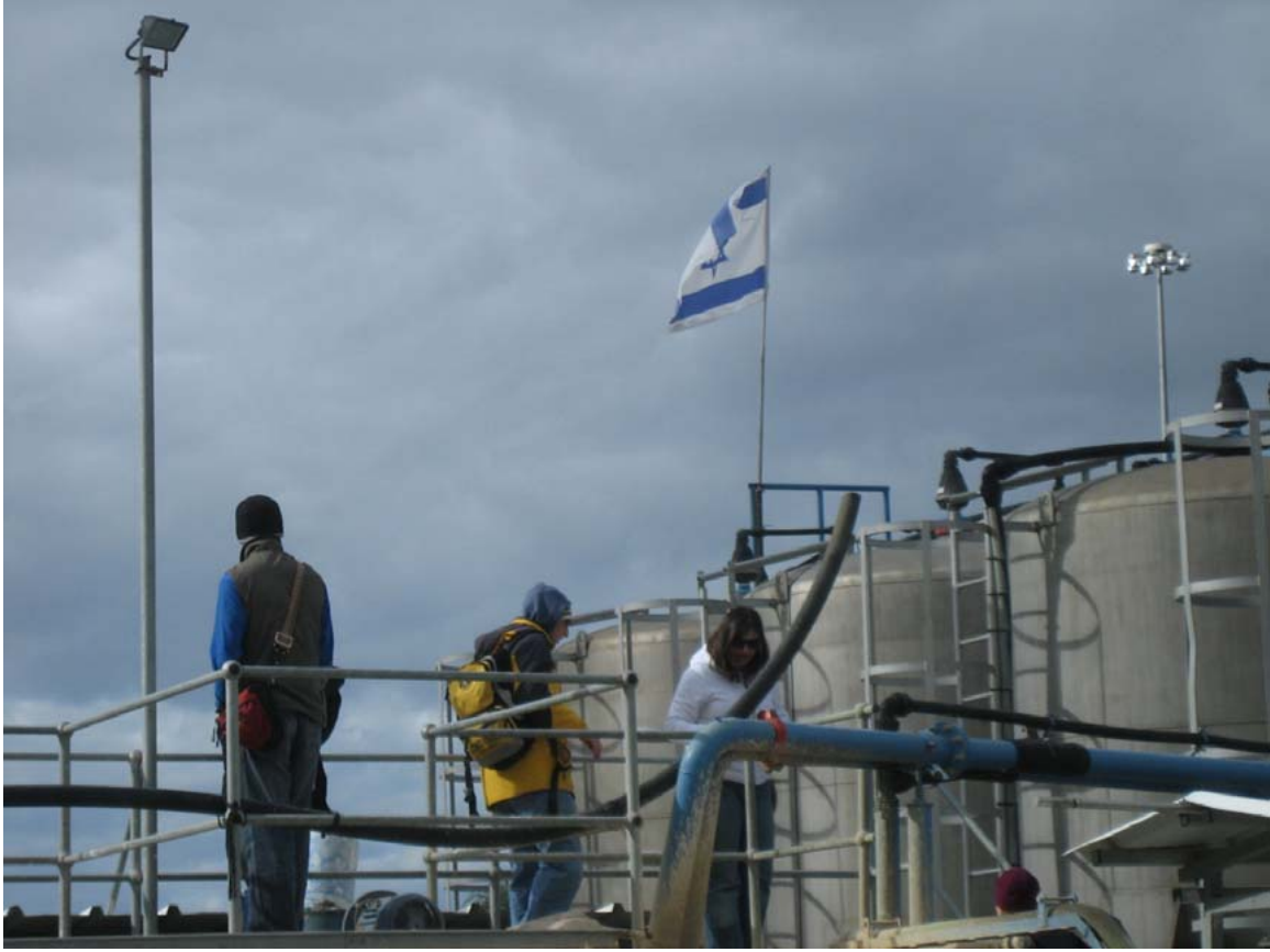
Figure 3: Yad Hana water treatment plant
