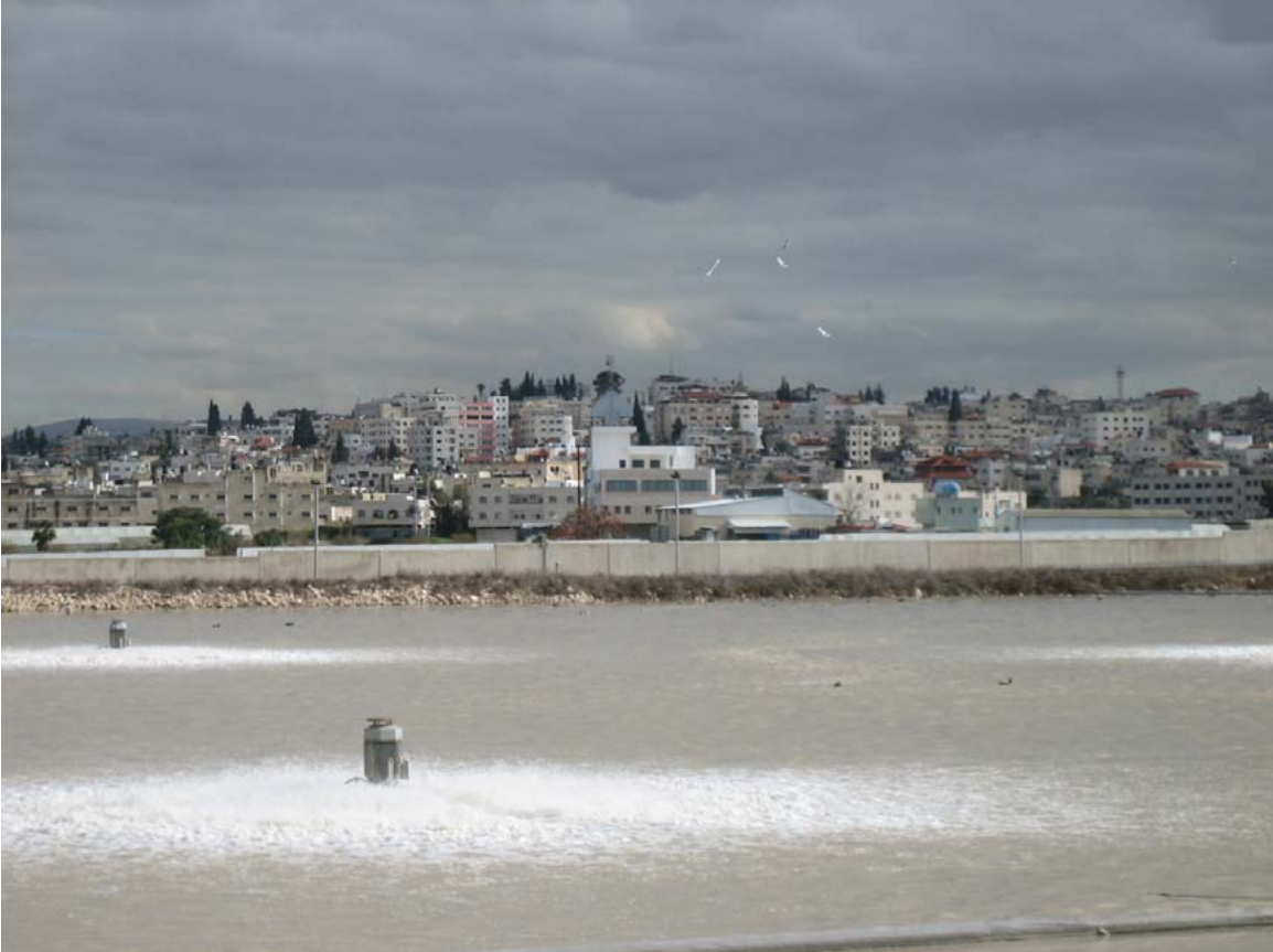
Figure 1: View of Tul Karm from Yad Hana water treatment plant
